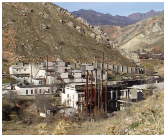
In harm’s way. The Isolite factory, a former uranium mill, is in line for a direct hit from a landslide.
